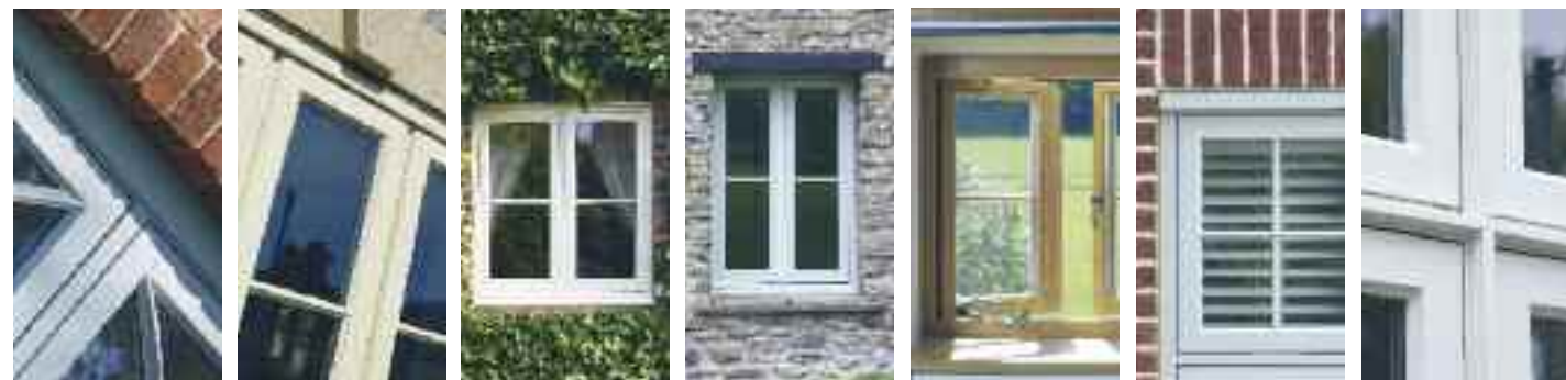
Flush Lipped Fixed mullion Floating mullion closed Floating mullion open Head drip detail Deco strip detail
