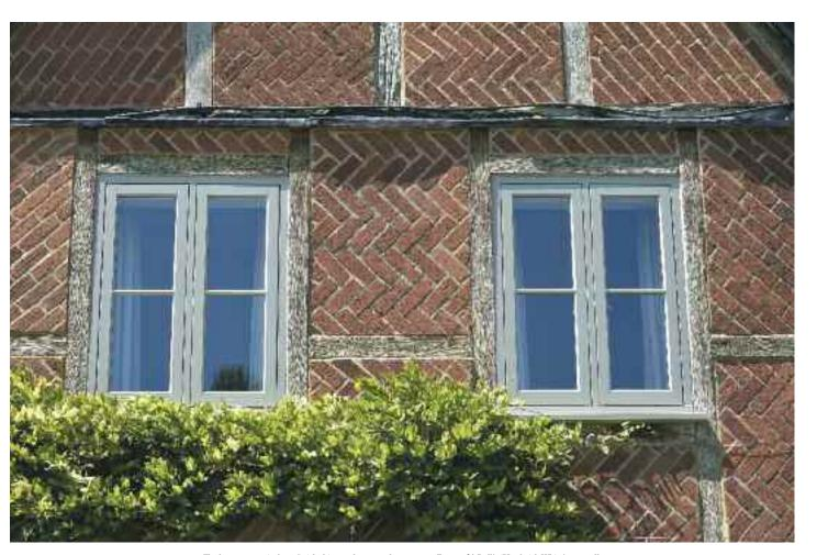
Flush casement windows finished in a colour complementary to Farrow & Ball's 'Hardwick White' externally and 'Ammonite' internally with 24mm true bars, putty glazing and 14mm ultra slim double-glazed units.
