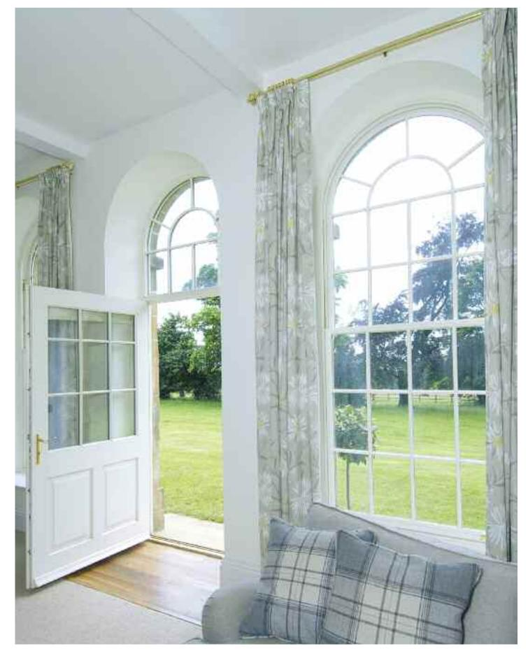
The new sash windows had to match the style and formation of the glazing bars from the original windows, the frames of which were still present once the openings were revealed.
