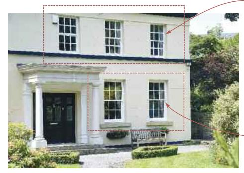
Existing replacement windows, Note: the thicker through bars, and incorrectly sized meeting rails and bottom
