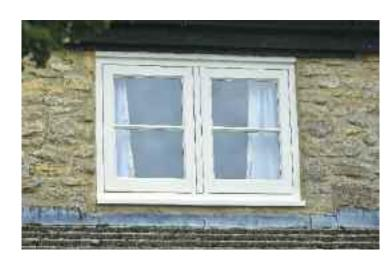
Replacing dark brown coloured windows, Mrs Grant opted for flush casement windows in a colour complementary to Farrow & Ball 'Pointing', a subtle, off-white shade. A simple horizontal 24mm true bar adds detail while 14mm ultra slim double-glazing units with traditional putty glazing, bring comfort and warmth.
