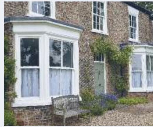
Slim sash windows in 'White', manufactured in Engineered European Redwood with 18mm astragal glazing bars.
