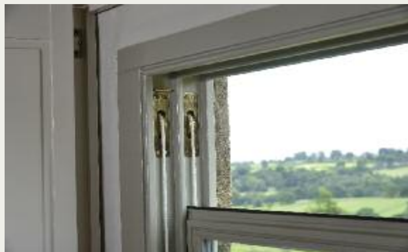
Slim sash windows with traditional cords & weights, finished in a colour complementary to Farrow & Ball 'Hardwick White' with 36mm astragal glazing bars and Mottled Antique Brass hook fasteners and sash lifts.
