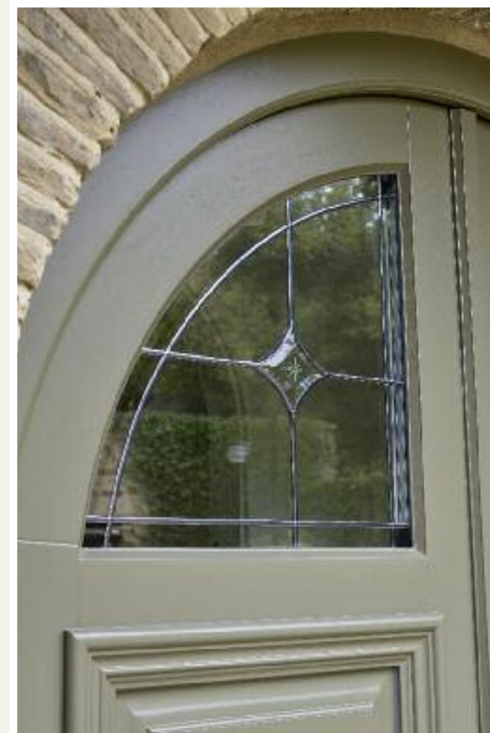
Bespoke, arched Hillingdon double entrance door finished in 'Oxford Clay' with Bevel leaded glazing design and an Antique Brass Unlacquered Profile Shoulder handle from Samuel Heath. Manufactured in Engineered Meranti Hardwood.
