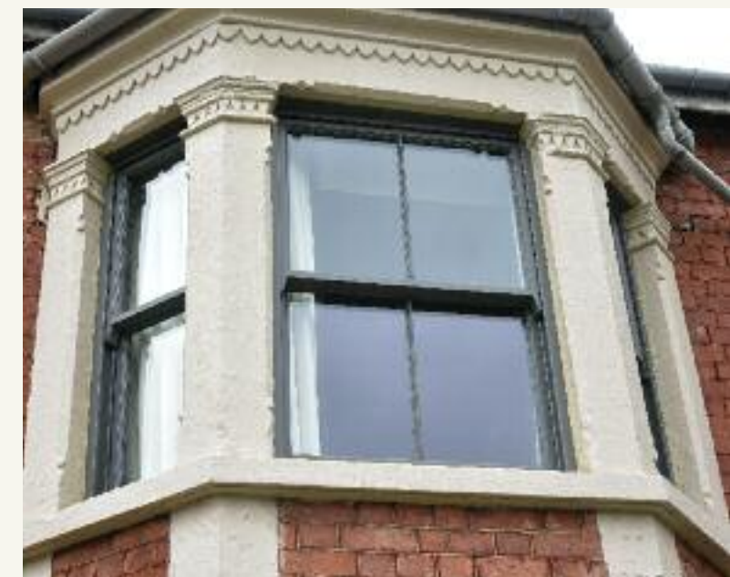
Slim sash windows finished in 'London Grey' with decorative sash horns including variations with vertical 18mm astragal glazing bar.
