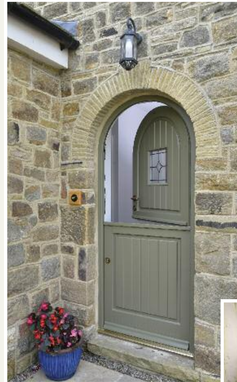
Staverton stable door finished in 'Oxford Clay' with Bevel leaded glazing design on 'Kathedral' patterned glass and an Antique Brass Unlacquered Extended Profile handle from Samuel Heath. Manufactured in Engineered Meranti Hardwood.
