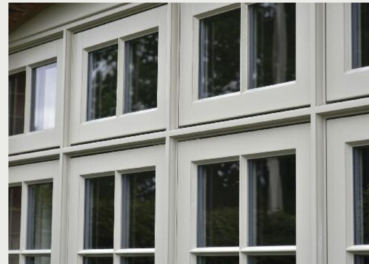
Deco casement windows finished in 'French Grey', with 18mm astragal glazing bars and manufactured in Engineered Meranti Hardwood.
